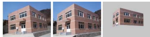
(a)Two original images of a building and a view of the reconstructed 3D surface
