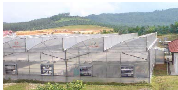
Fig. 5: Greenhouse with four ventilation fans and planting troughs inside
