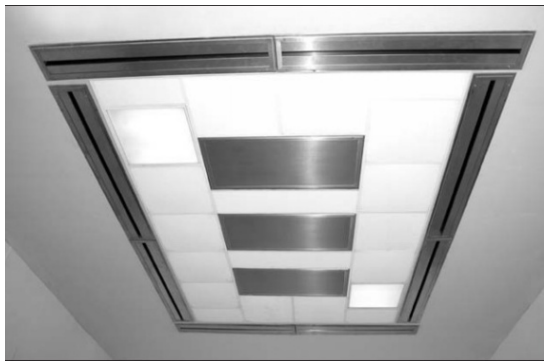
Figure 6- The layout of vertical laminar airflow system with the air curtain
