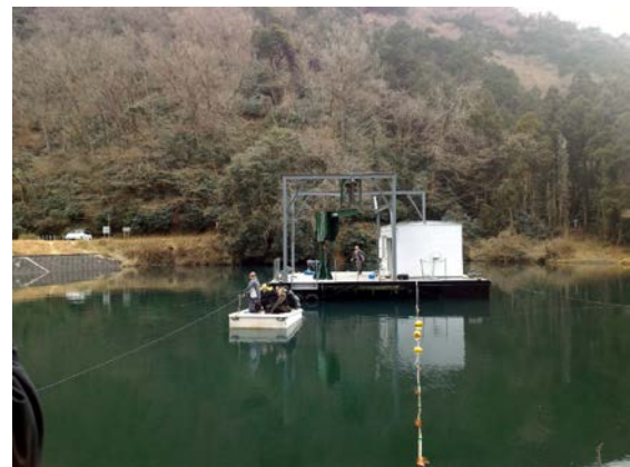
Fig. 11: Floating Barge in Nagase Dam
