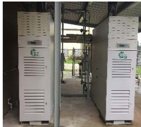
Fig. 10(a) Snapshot of deployed camera images of MG critical assets (a) two CHP generator
