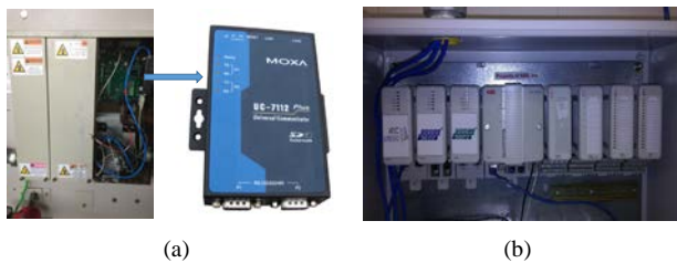
Fig. 4 (a) Communication bay of Capstone microturbine including modbus translator and (b) DCS 800XA showing IO and communication module.
