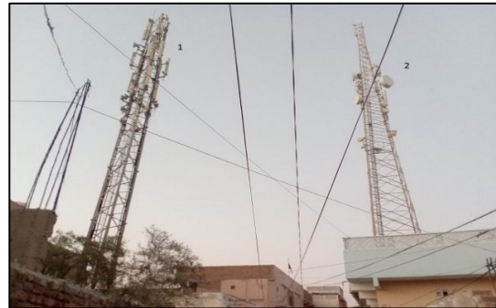
Fig.2. Two BTS operators on the same location
