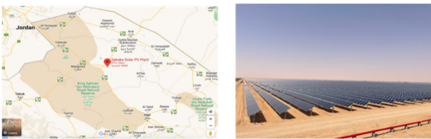
Fig. 1 IPP photovoltaic plant, Sakaka, Saudi Arabia.
