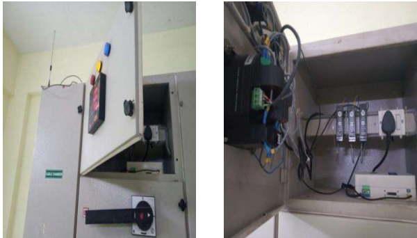
Fig.7. Hardware installation of energy monitoring system using GSM gateway
