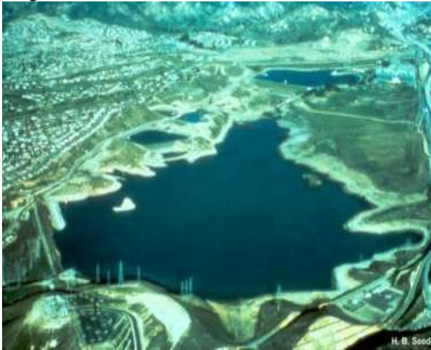
Figure 1: A bird eye view of San Fernando dam and its reservoir.
